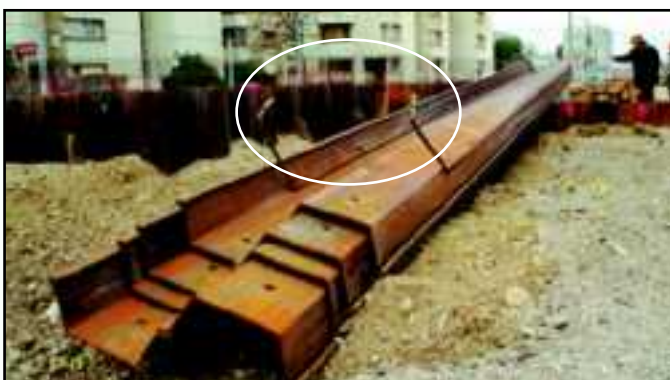
The top of the jetting pipe may be bent to facilitate connection of the supply hose.
