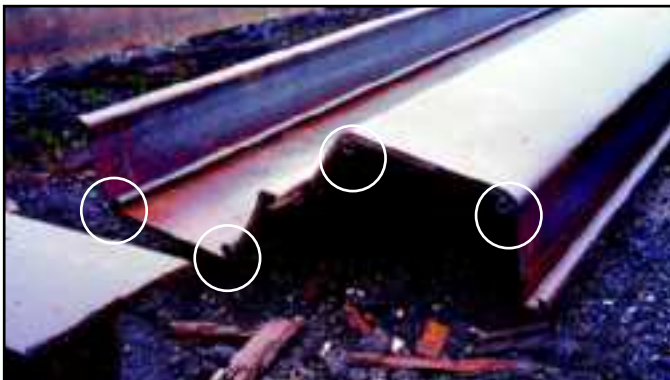
The jetting pipe ends flush with the toe of the sheet pile.
