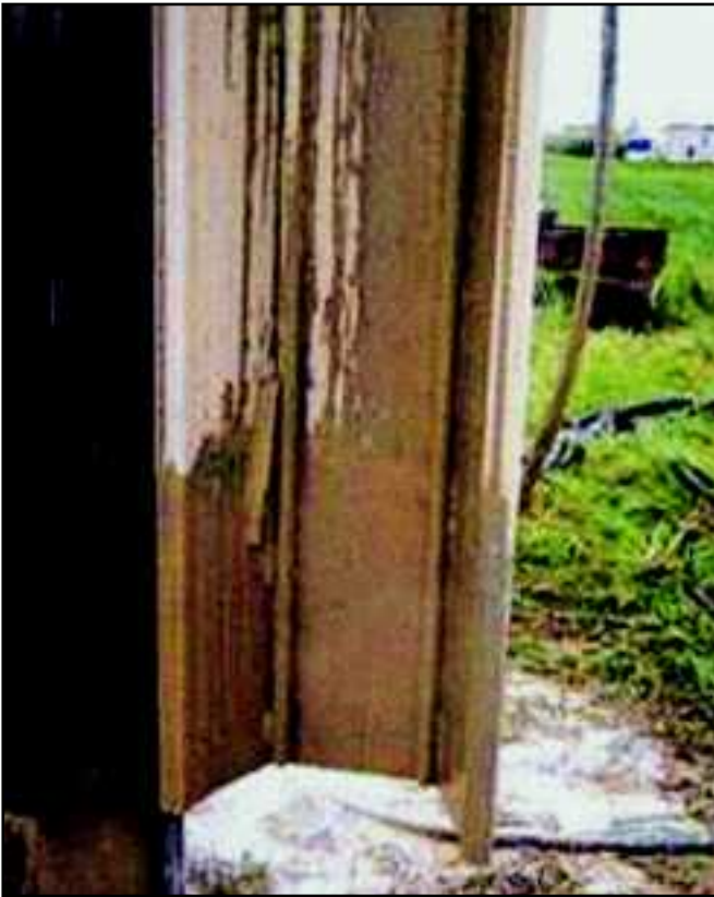
Photo 2: Extracting jetted U pile
