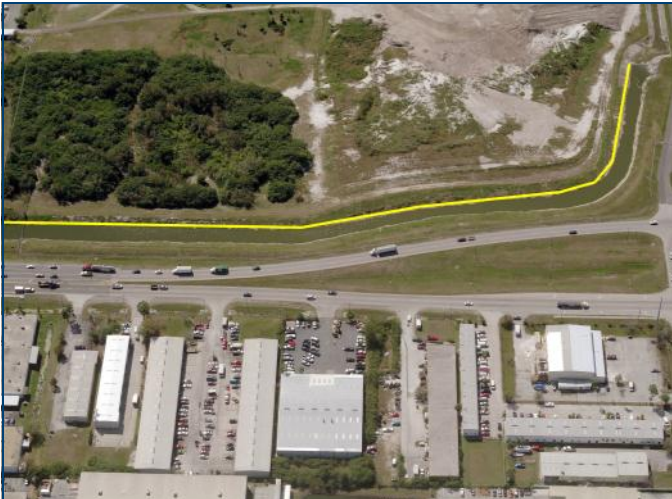
"(The sheet pile wall with hydrophilic sealant) results in a permeability of less than 5 \times 10^{-11} cm/sec." - SCS Report
