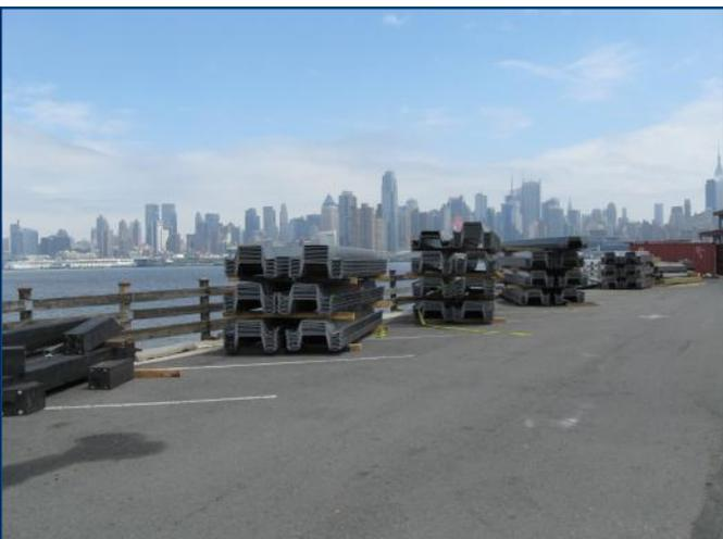
UC-50 is a 36" wide "box" shaped profile which greatly reduced the amount of interlocks on the face of the wall.
