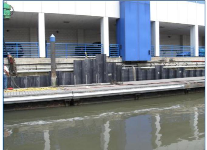
The sheets varied from 15' to 30' long and were driven into various soil conditions at an average of 100 feet per day.
